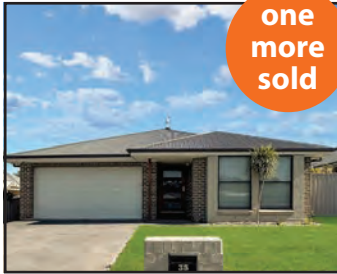
35 Hewitt Avenue, St Georges Basin
